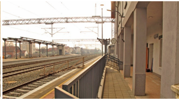
Figure 15. New railway station Doljevac (Z. Cvetković, 2025)
