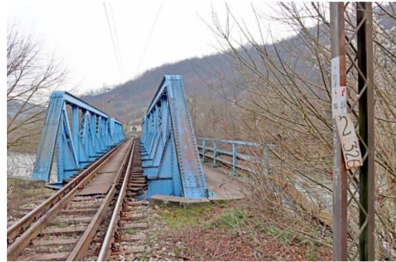
Figure 7. Lepenica Bridge over the South Morava River, (Z. Cvetković, 2025)
