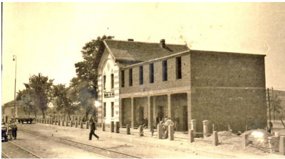
Figure 14. Railway station Doljevac built in 1886, (source: Wikimedia)
