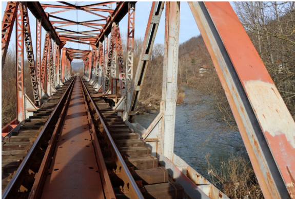
Figure 6. Grdelica Bridge over the South Morava River, (Z. Cvetković, 2025)
