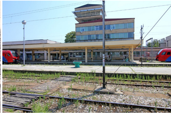
Figure 9. New railway station Niš (Z. Cvetković, 2025)
