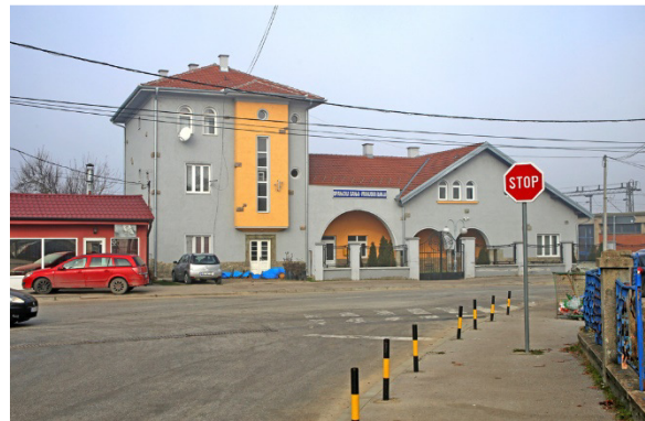
Figure 30. Railway station Vranjska Banja, (R. Kulenović, 2025)
