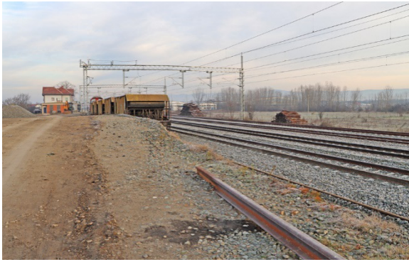
Figure 12. The railway reconstruction at the station Belotinac(Z. Cvetković, 2025)
