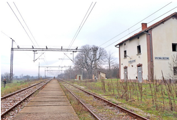
Figure 18. Railway station Brestovac (Z. Cvetković, 2025)
